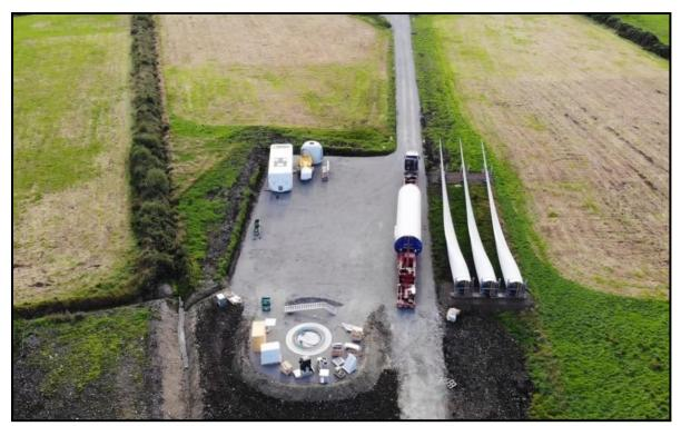
Plate 10. Example of typical finished hardstand on a wind farm.
